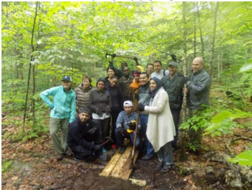
Building a Bog Bridge at Brewster Peninsula
